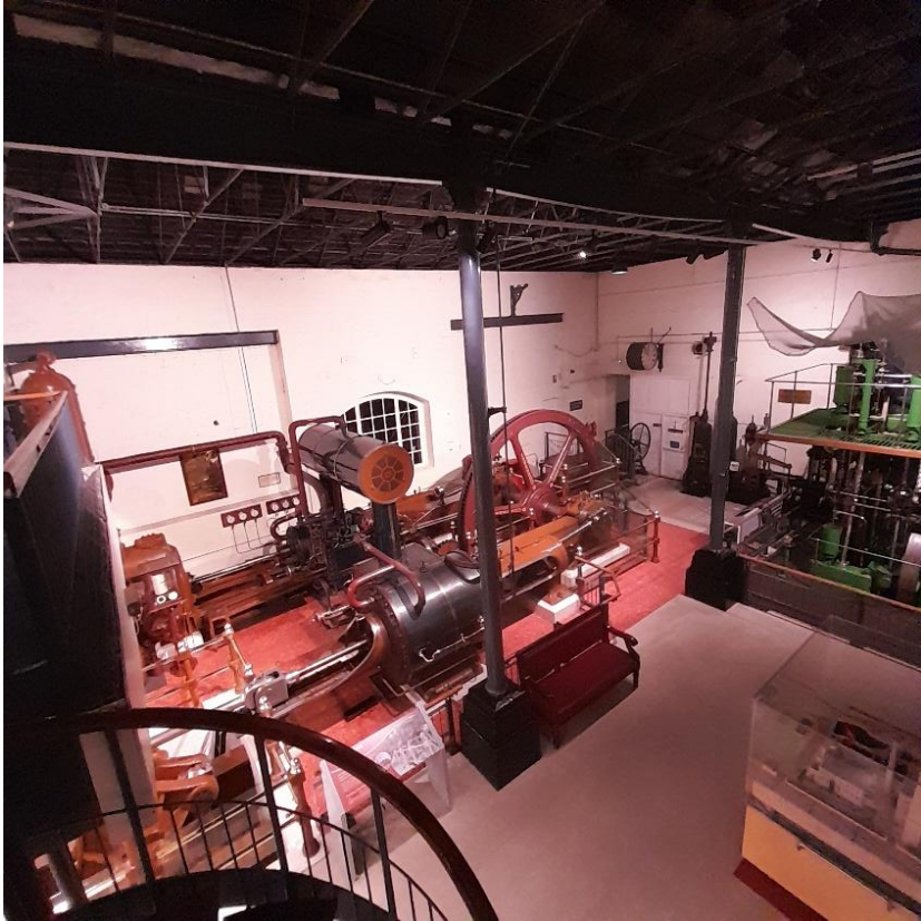
WADDON PUMPING STATION ENGINE (1)
