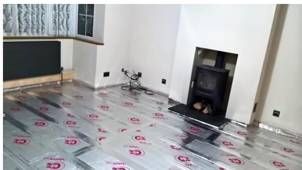
Underfloor insulation using Celotex
