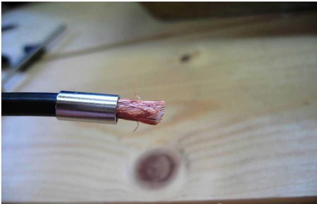
Make sure you have the crimp sleeve in place – especially if this is the second connector on a length of coax.
